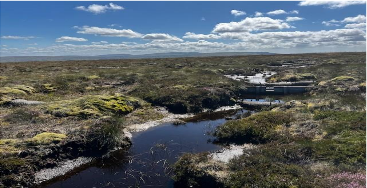
Plate 4.8 Timber dam/sediment trap installed at a restoration site in the Yorkshire Dales
