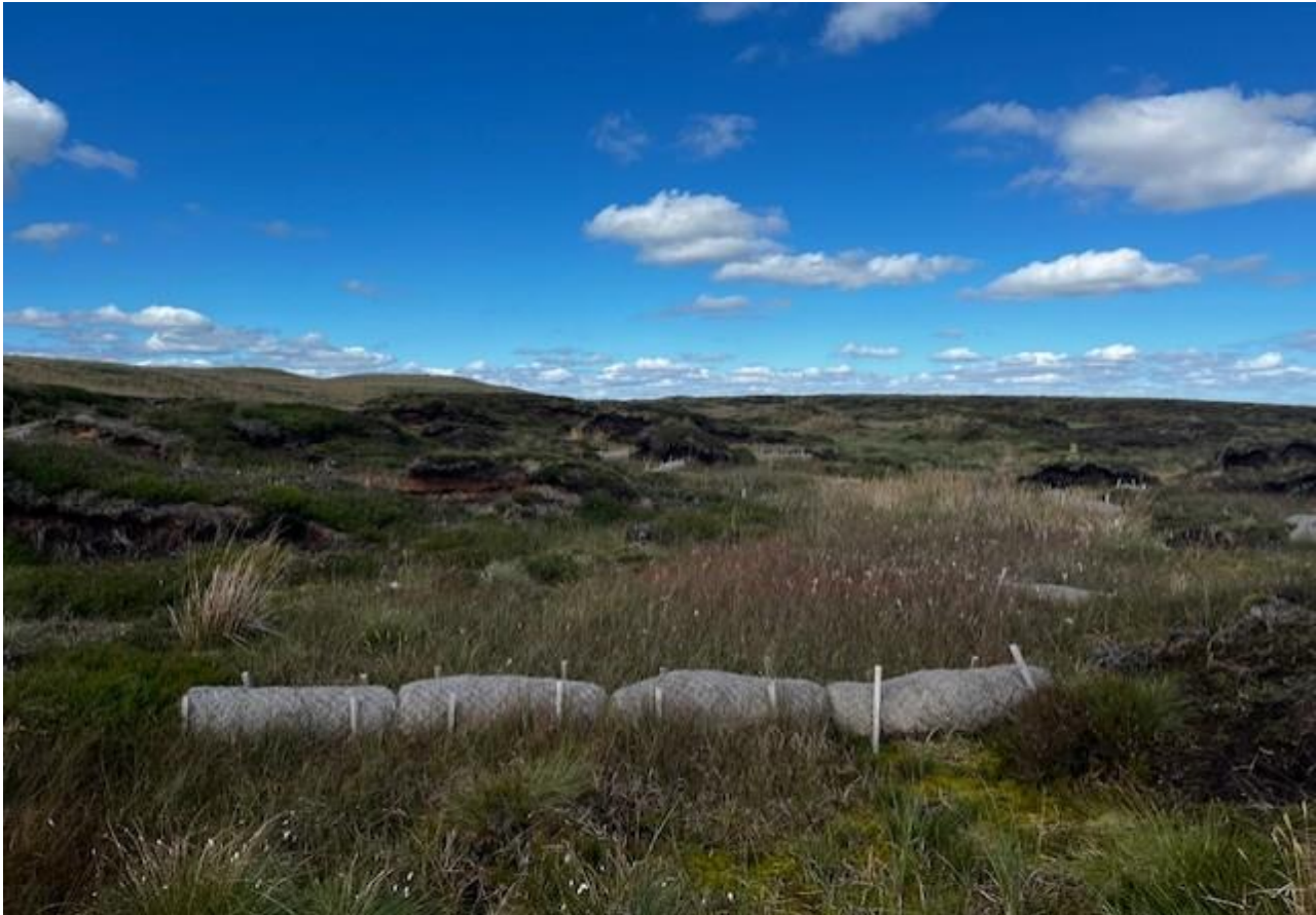
Plate 4.7 Example of gully bunds within revegetated peat filled gulleys at a restoration site in Yorkshire Dales
