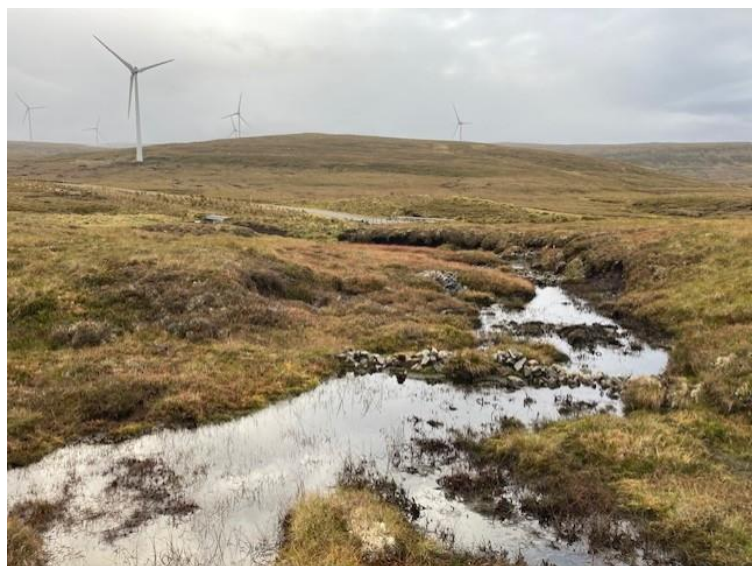
Plate 4.9 Stone dams within mineral/shallow peat gullies at a wind farm site in the Monadhliath mountains
