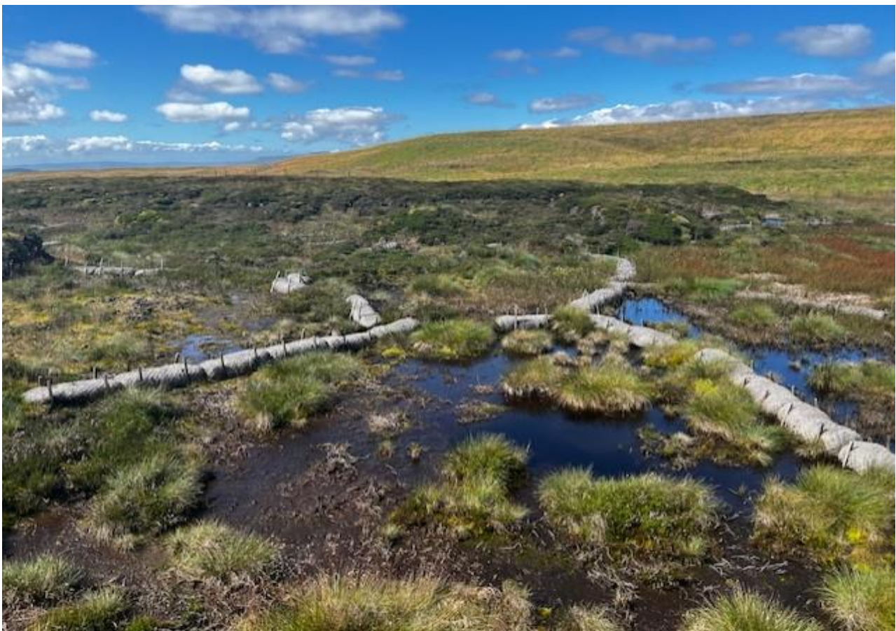
Plate 4.6 Example of cell bunding using coir rolls at a restoration site in Yorkshire Dales
