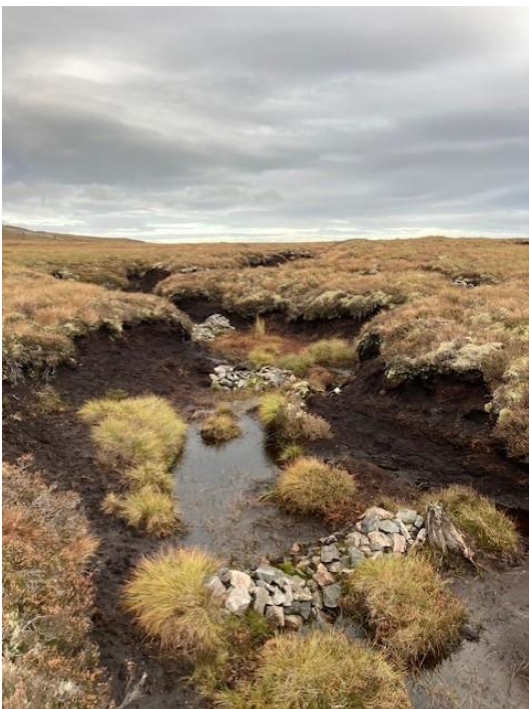
Plate 4.9 Stone dams within mineral/shallow peat gullies at a wind farm site in the Monadhliath mountains
