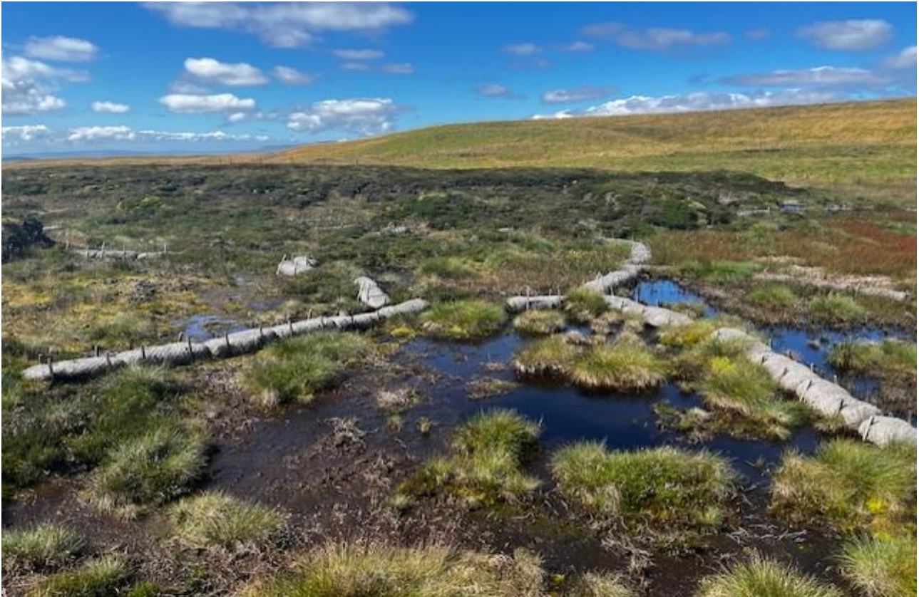
Plate 4.6 Example of cell bunding using coir rolls (restoration site in the Yorkshire Dales)
