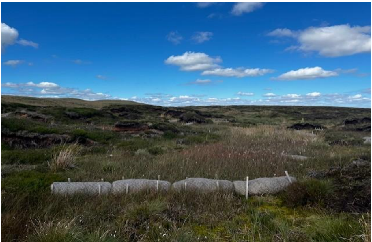
Plate 4.7 Example of gully bunds within revegetated peat filled gulleys ( restoration site in the Yorkshire Dales)
