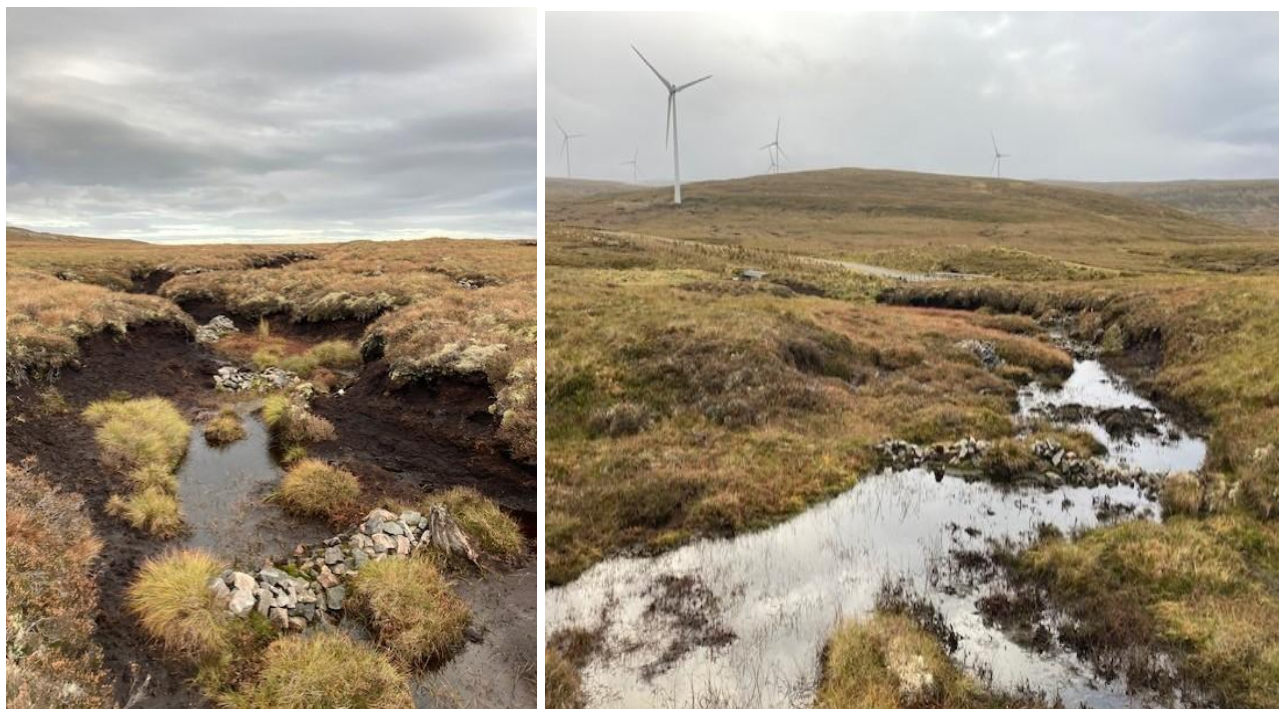
Plate 4.9 Stone dams within mineral/shallow peat gullies (site in the Monadhliath mountains)
